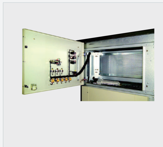
Figure 3/7 View of Low Voltage Compartment
